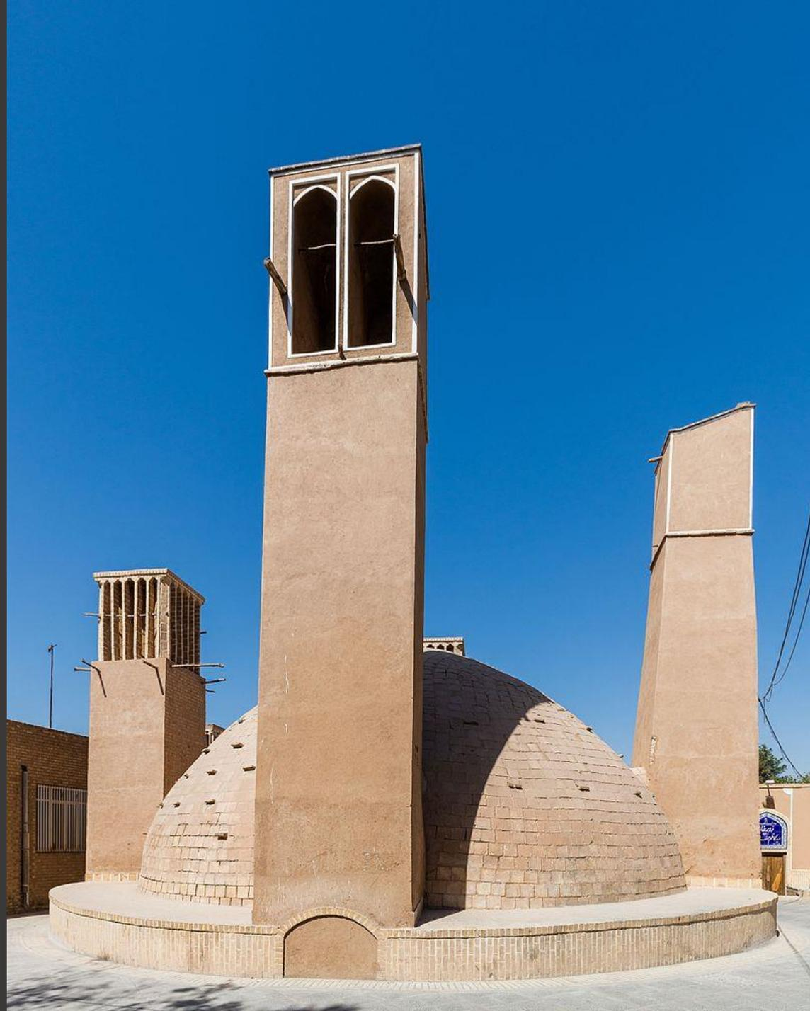
The shape of the tower, alongside factors like the layout of the house, the direction the tower is facing, how many openings it has, its configuration of fixed internal blades, canals and height are all finely tuned to improve the tower's ability to draw wind down into the dwellings below.
